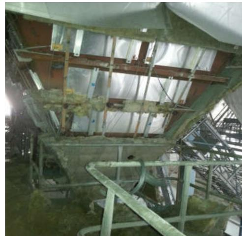
Fig.3 Stripped Insulation from a hopper
